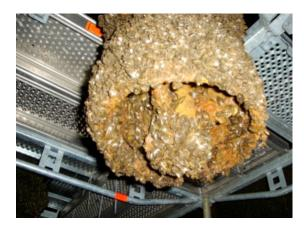
Bacteria thrive underneath the mussel colonies, and anaerobic respiration by these bacteria produces acidic compounds, that can accelerate corrosion and pitting of pipelines.
